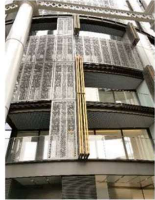
Source: Mayor of London. (2018). Energy, overheating and daylight in tall buildings study Old Oak and Park Royal Development Corporation, Buro Happold, for the Mayor of London.
