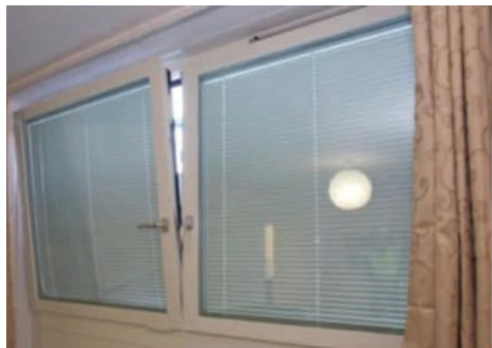
^ Installed windows with blinds drawn. (Permission United House).
