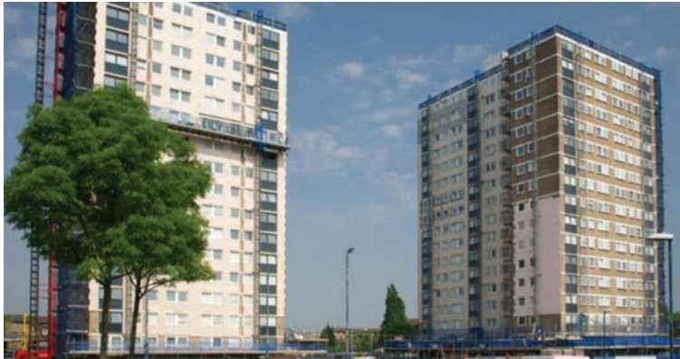
^ External cladding being applied (Permissions LBBB).
