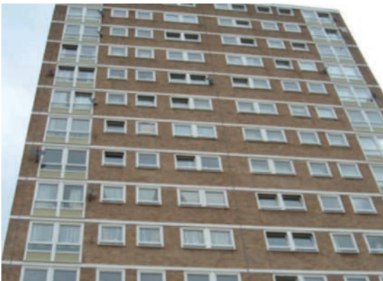
^ Outer finish of blocks before refurbishment (Permission of LBBB).
