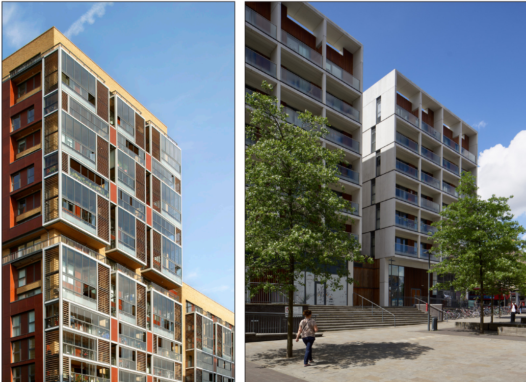
Figure 1 (left): Mitigating overheating risk with noise-attenuating sunspaces.
