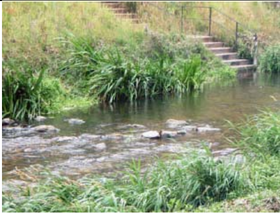
Provision of gravel/rock riffles within the channel
